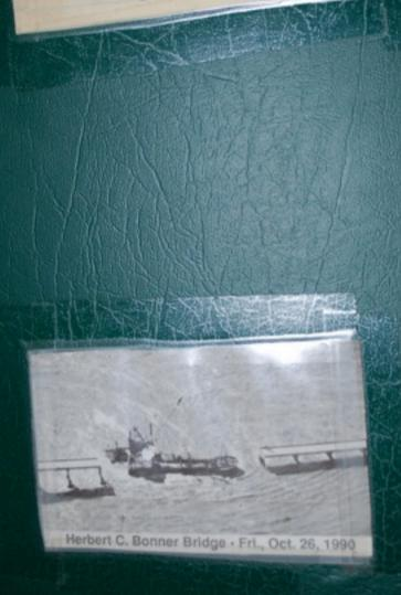
On October 26,1980 a dredge was driven by a terrific rain and wind storm into the Herbert Bonner Bridge across Oregon Inlet. It knocked out 370' of bridge and cut off Hatteras Island from the northern beaches and the mainland. The island was left without power and telephones.
