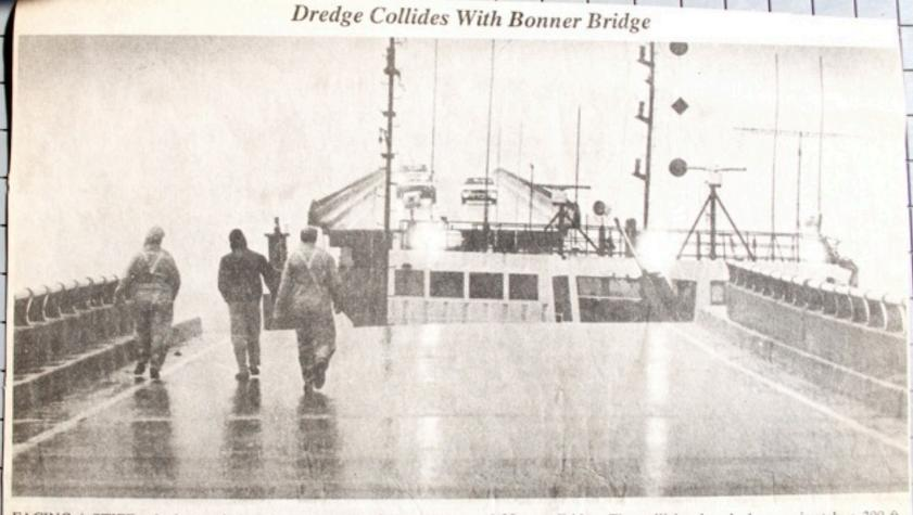
FACING A STIFF gale-force wind, three county officials carefully make their way to the spot where the dredge Northerly Isle crashed into the Herbert C. Bonner Bridge, spanning Oregon Inlet at about 1:30 a.m. Friday. The collision knocked approximately a 300 ft. section from the north end of the bridge, closing the structure to all traffic for an undetermined length of time. (J. Wooten photo)
